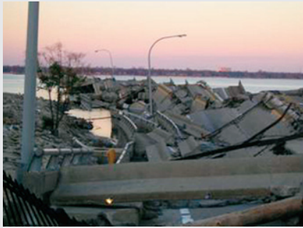
Source: GAO. U.S. 90 Bridge in Biloxi, Mississippi.
